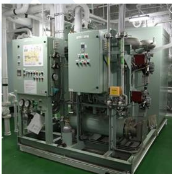
Figure 1.13 Membrane N 2 Generator System (Courtesy of Kashiwa Co., Ltd.)
